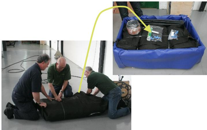
Once unpacked all that is required is a few simple steps and the Flexigester can be ready for use within a day. The installation needs only simple hand tools, no power and no waiting for concrete or cement to set.
